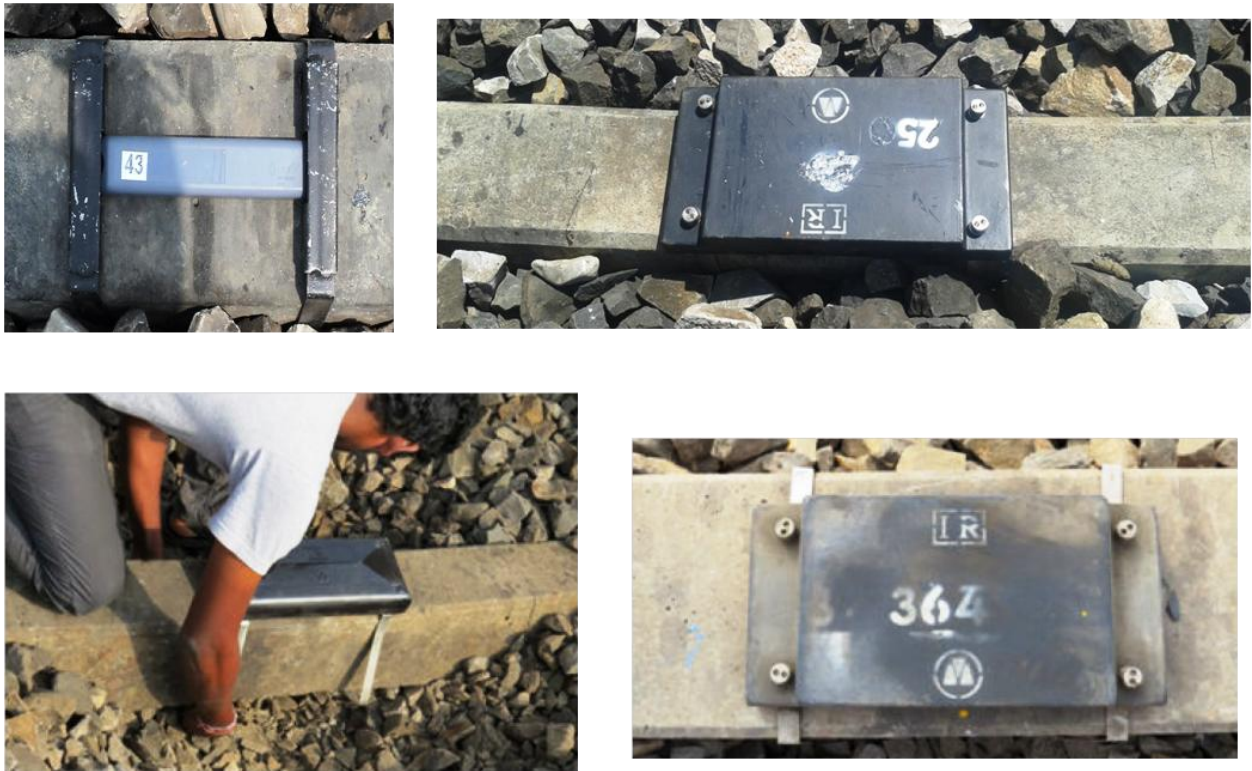
Figure 36: RFID Tag installation
